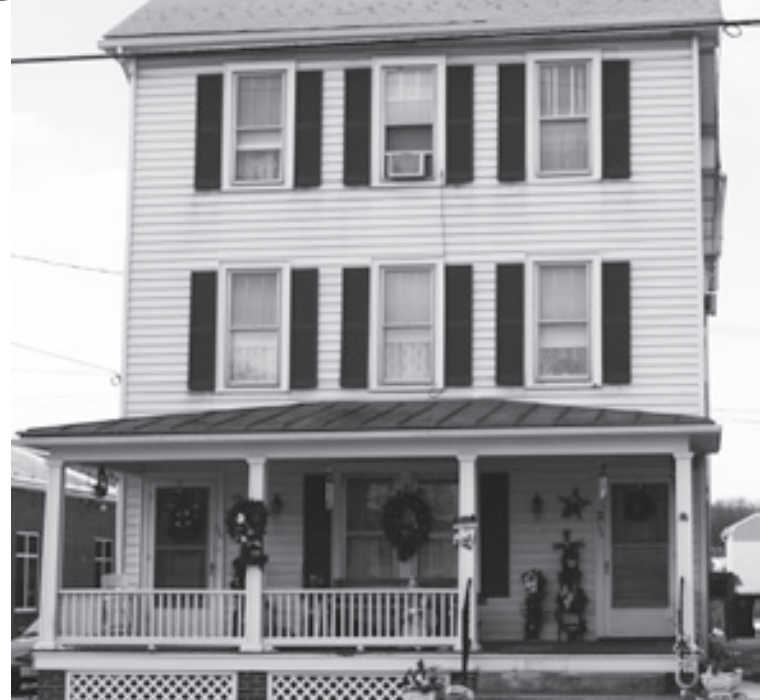
In the 1940's the old Emerald Building was bought by John Hollinger, who converted the two-story structure into its present three-story layout by removing the original 12 foot high ceiling and replacing it with two 8 foot floors.
