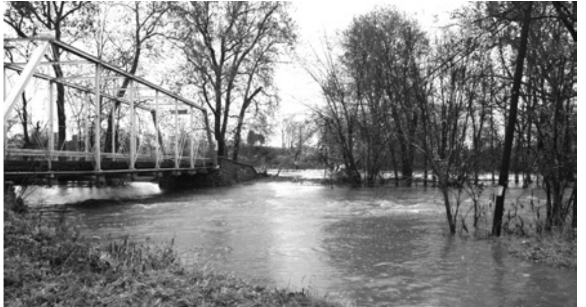
A good gage of the severity of a storm is the height of the water under Toms Creek Bridge.
