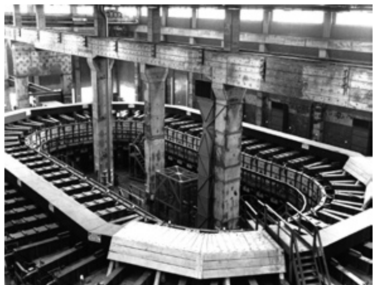
K-25 used gaseous diffusion to enrich uranium from Fernald by separating uranium-235 from uranium-238.
