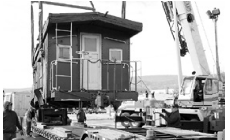
The Cozy caboose being loaded on a trailer for its trip to its new home in Virginia.
