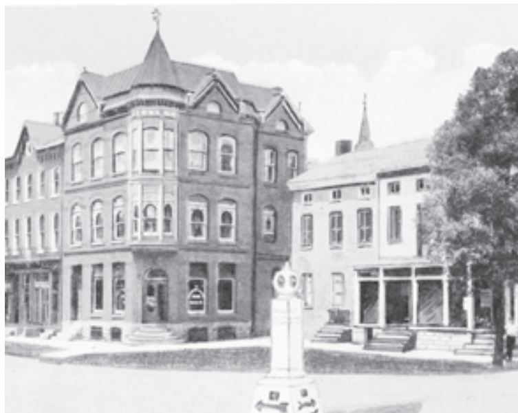
At one time, the Banking House of Annan-Horner was the most eye-catching and prestigious building on the square: fitting for the leading role it played in the development of Emmitsburg in the early 1900s.
