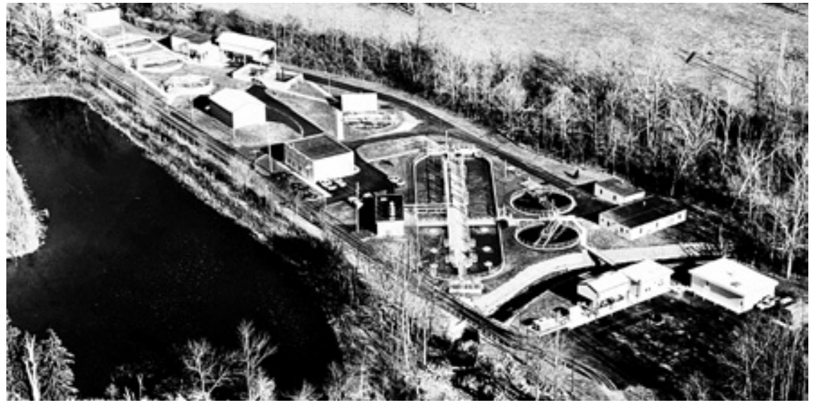
Thurmont's waste water treatment facility.
